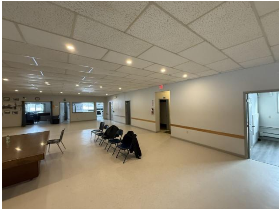
Photo 3: Recreation Hall – Overview of Interior Finishes
