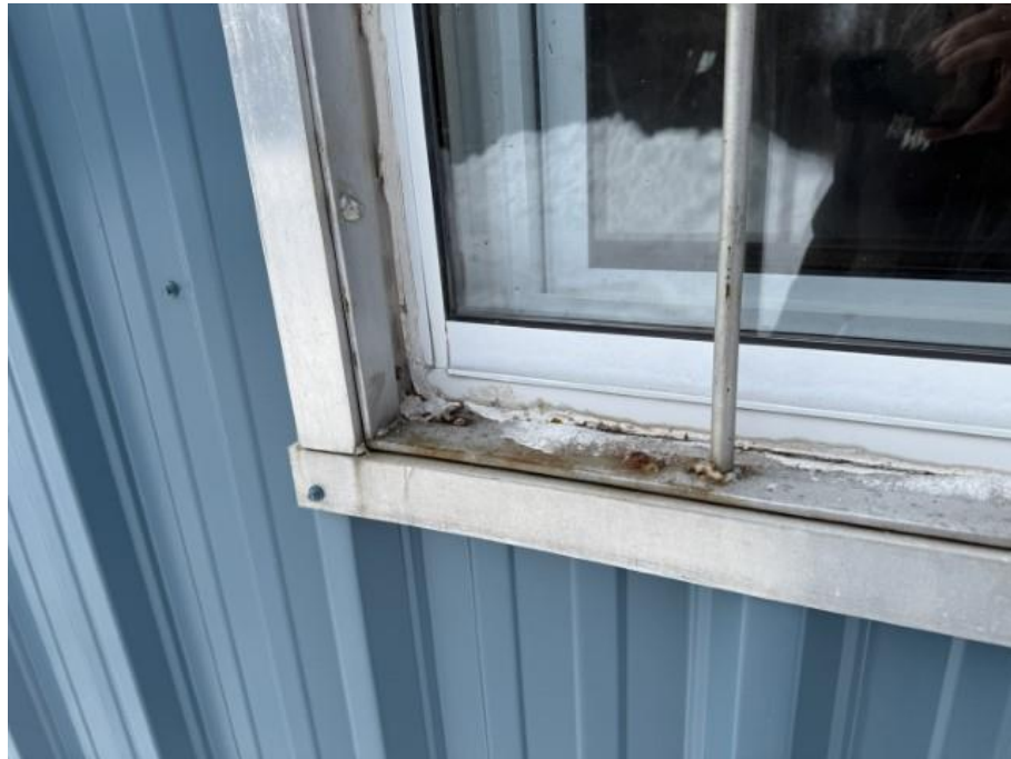
Photo 9: Municipal Garage – Overview of Exterior Windows and Sealant
