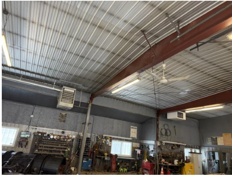
Photo 5: Municipal Garage – Overview of Steel Structure
