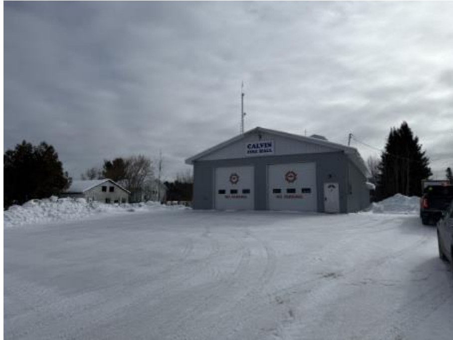
Photo 1: Fire Hall - Overview
