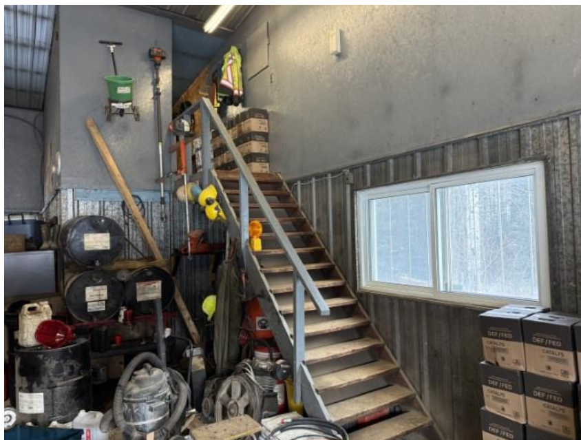
Photo 6: Municipal Garage – Wood Framed Loft Structure
