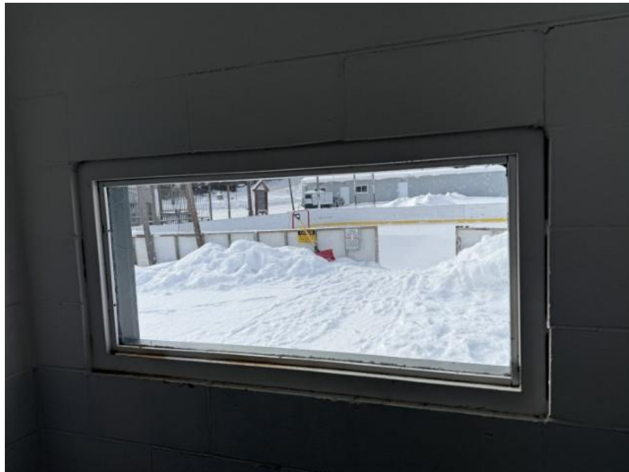
Photo 6: Changing/Storage Building - Windows
