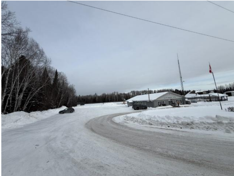
Photo 1: Main Parking Area
