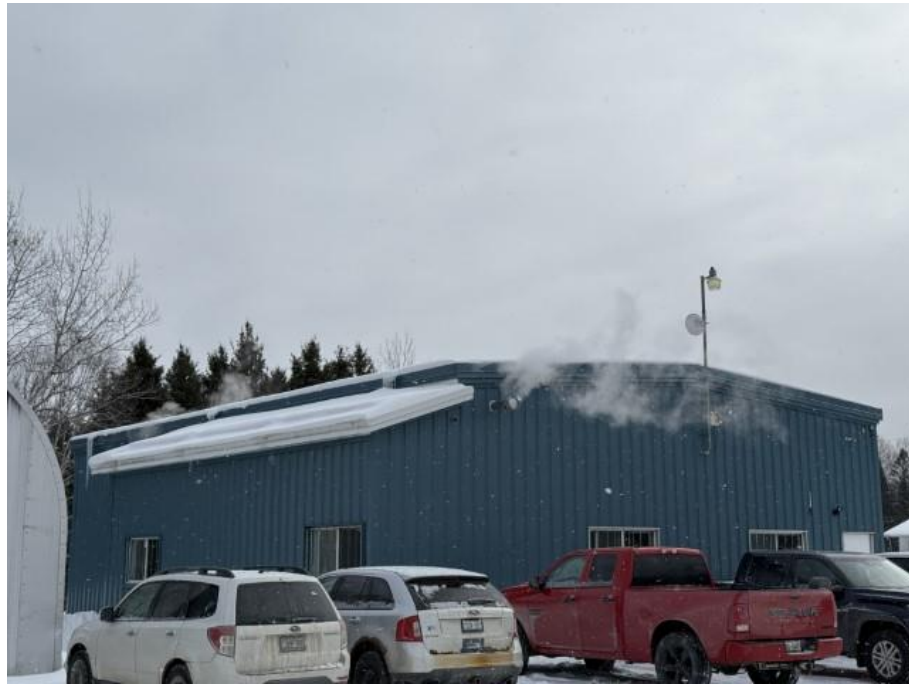
Photo 13: Municipal Garage – Overview of Covered Roof
