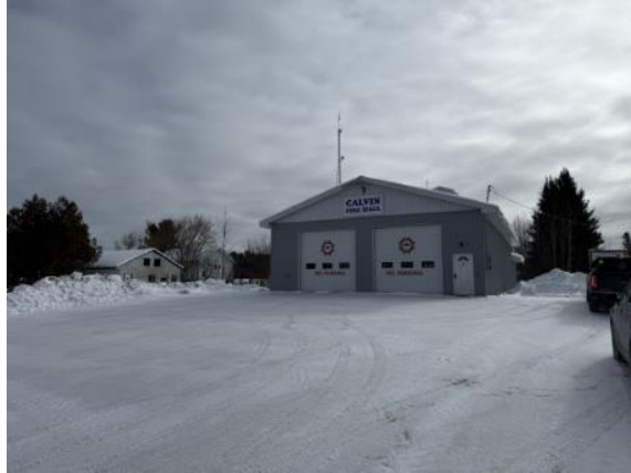
Figure 2. Overview of Fire Hall Building
