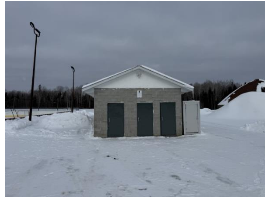
Figure 7. Overview of Equipment Building
