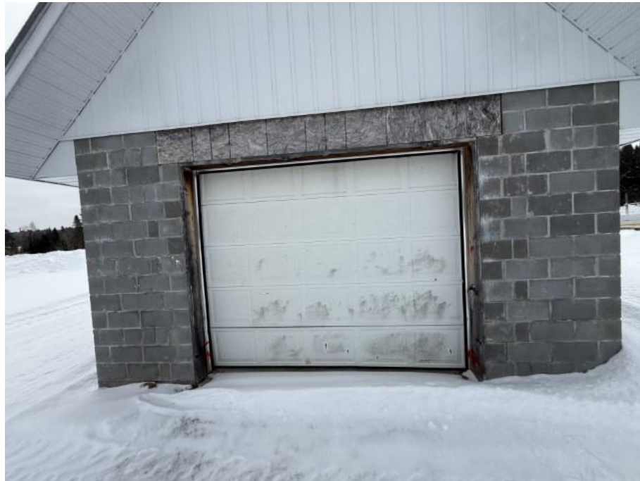
Photo 7: Changing/Storage Building – Garage Door
