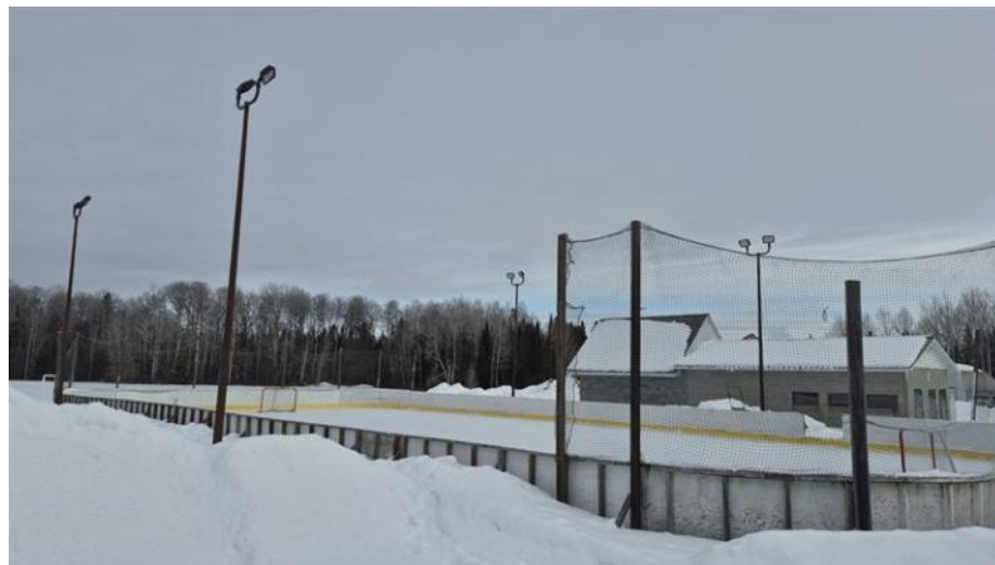
Photo 10: Ice Rink – LED Floodlighting
