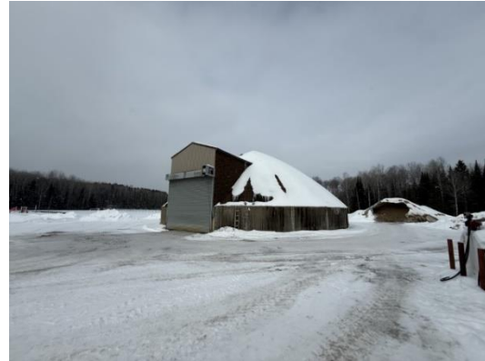
Figure 3. Overview of Sand Dome
