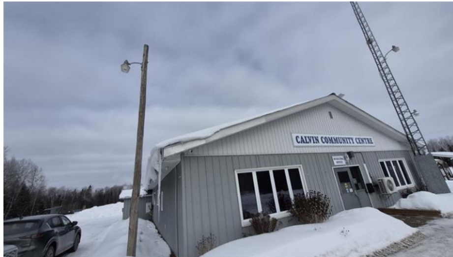
Photo 21: Recreation Hall – Existing HID Exterior Lighting
