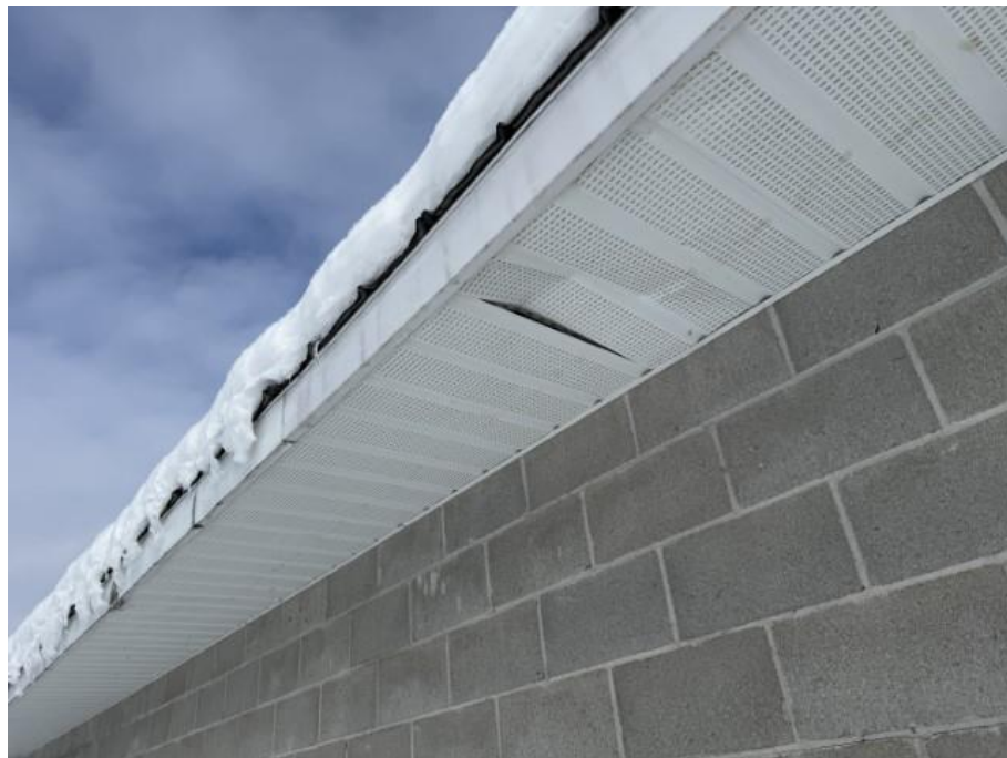
Photo 8: Changing/Storage Building – Metal Soffit
