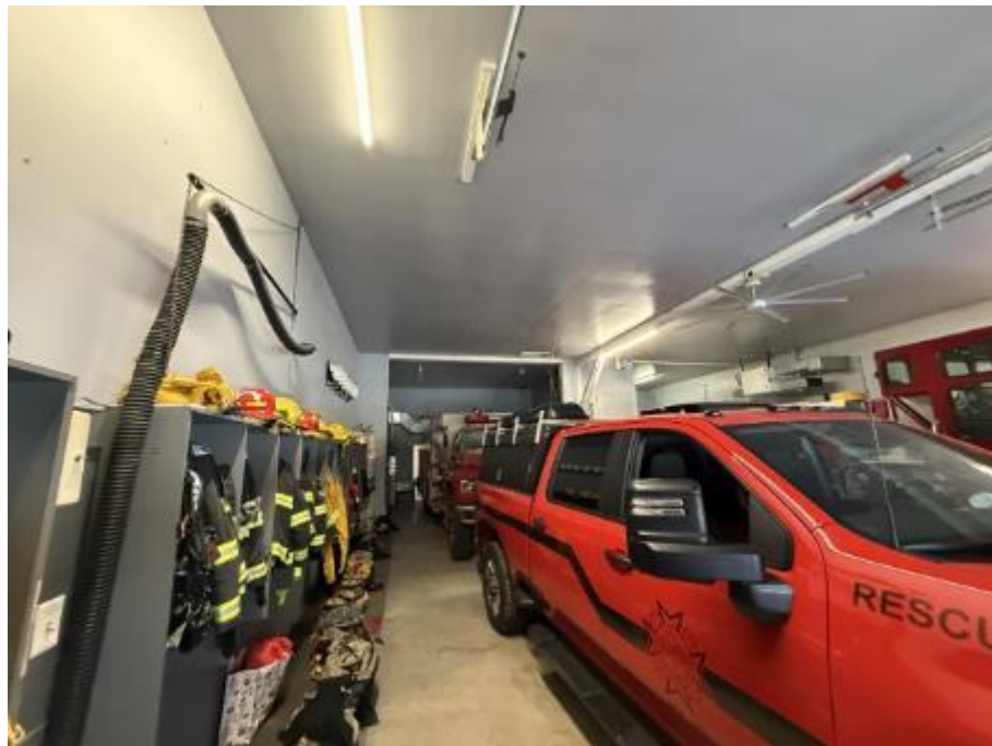
Photo 4: Fire Hall – Overview of Interior Finishes and Existing Vehicle Exhaust Tube
