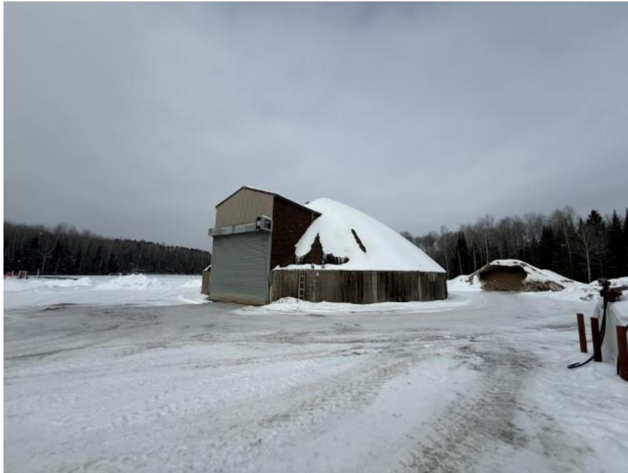
Photo 1: Sand Dome –Overview
