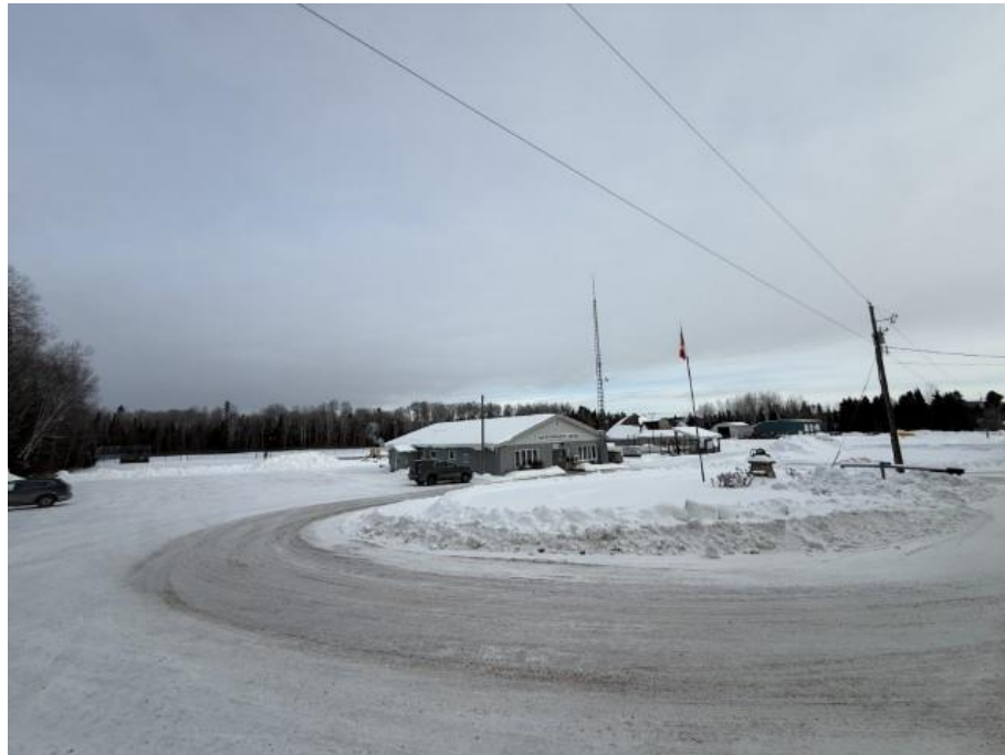
Photo 11: Recreation Hall – Overview of Covered Roof
