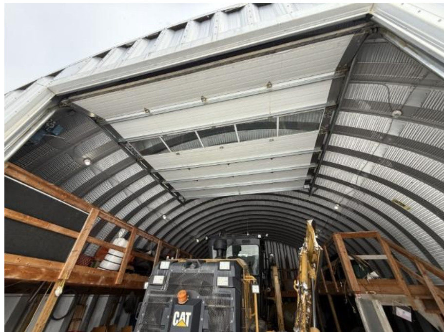
Photo 8: Quonset Hut – Overhead Door
