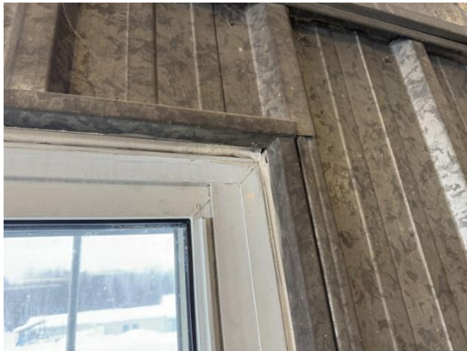
Photo 10: Municipal Garage – Overview of Interior Sealant
