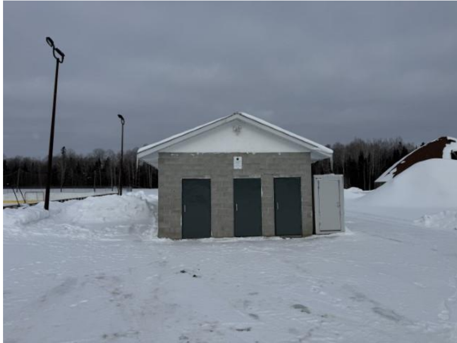
Photo 1: Changing/Storage Building - Overview
