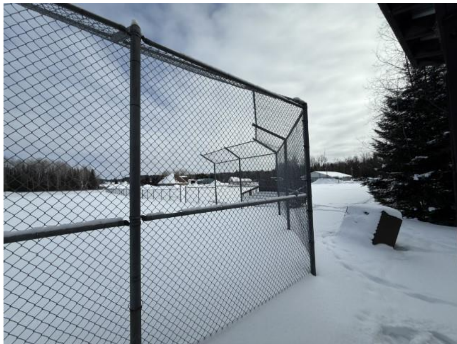
Photo 6: Overview of chain Link Fence
