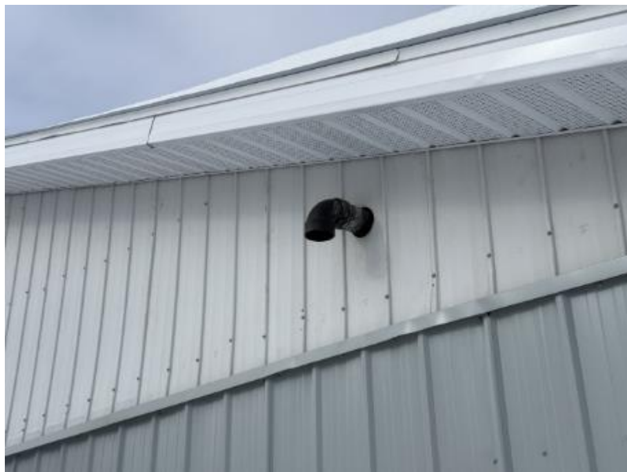
Photo 6: Fire Hall – Typical Penetration
