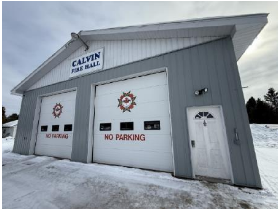
Photo 8: Fire Hall – Typical Garage and Man Doors
