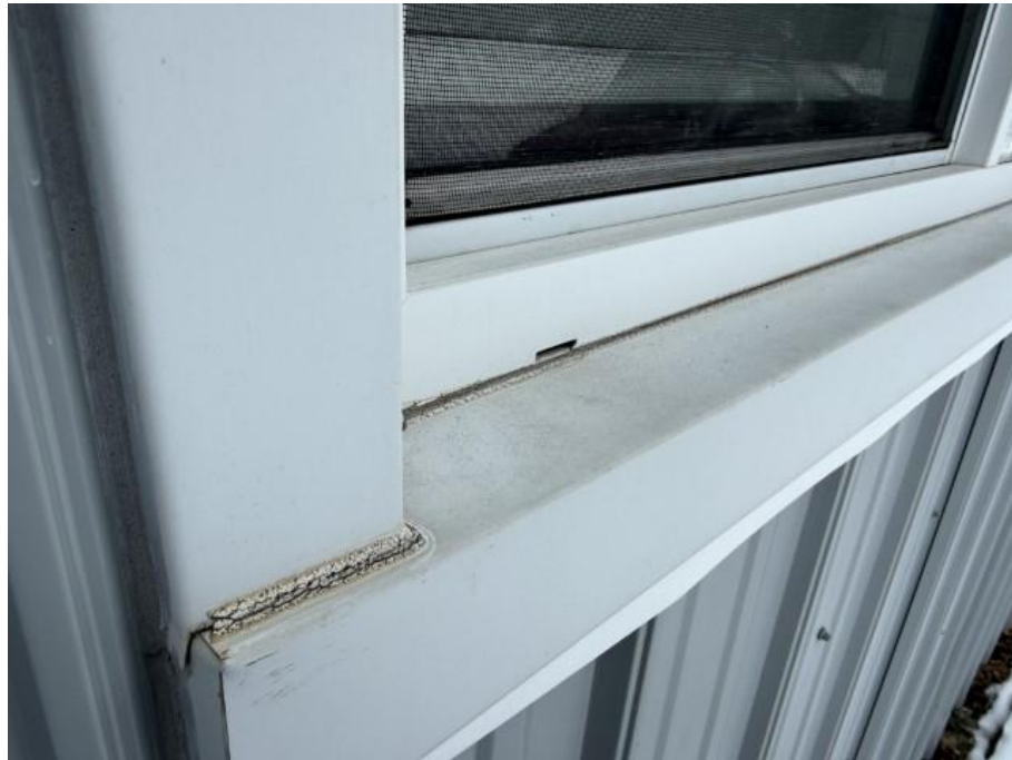
Photo 7: Recreation Hall – Windows and Sealant Exterior
