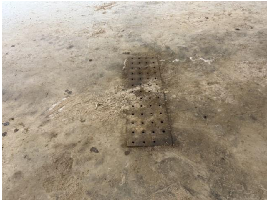
Photo 4: Municipal Garage – Typical Slab Drain
