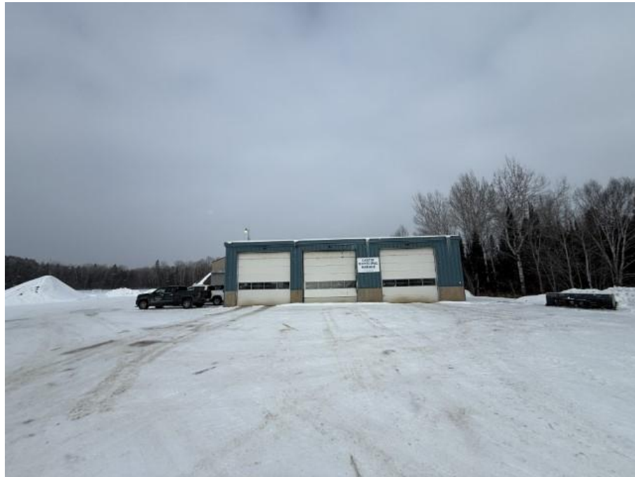
Photo 1: Municipal Garage – Overview of Building
