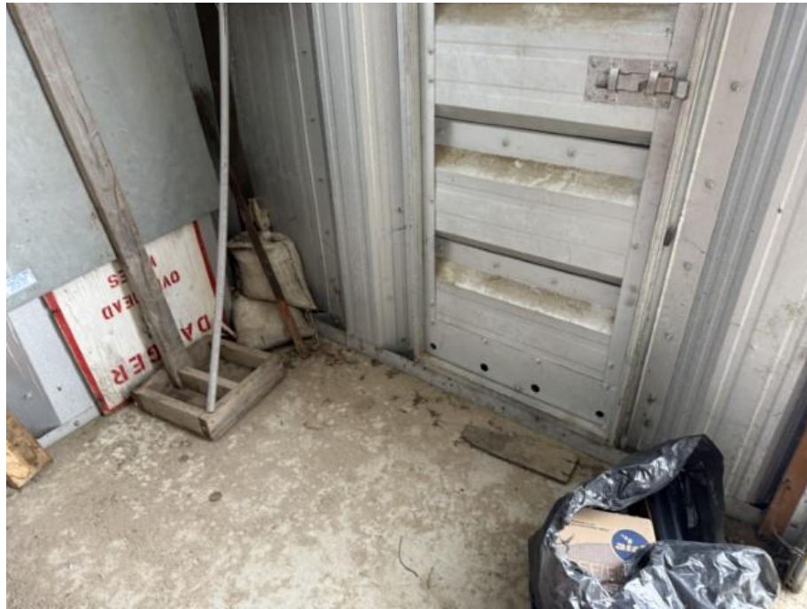
Photo 7: Quonset Hut - Man Door
