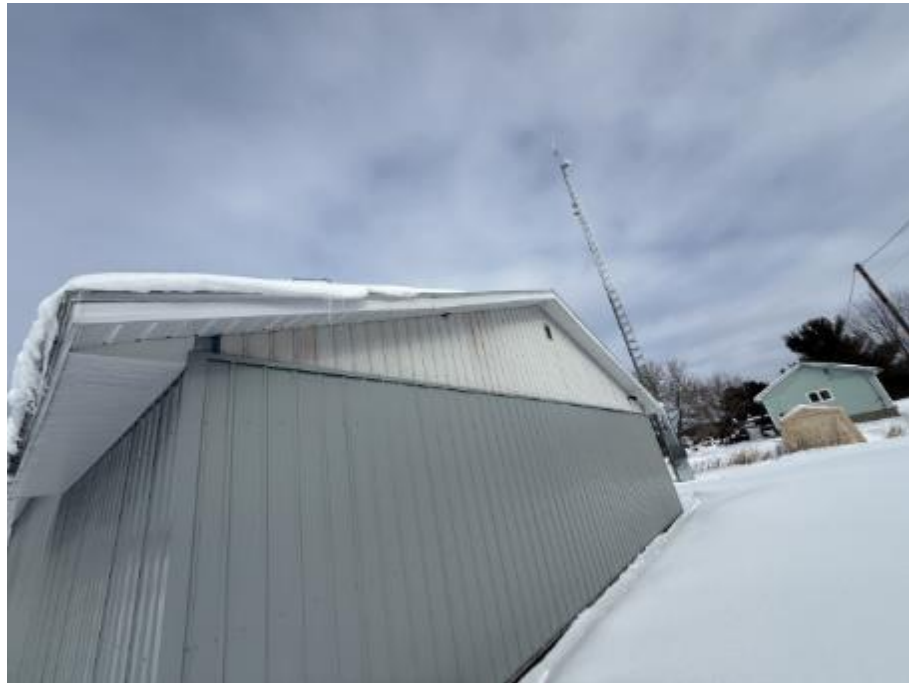
Photo 5: Fire Hall – Overview of Two Vintages of Siding
