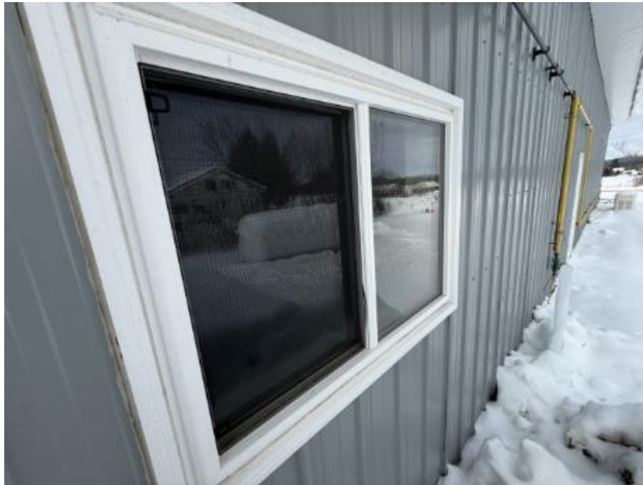
Photo 7: Fire Hall – Typical Windows and Sealants
