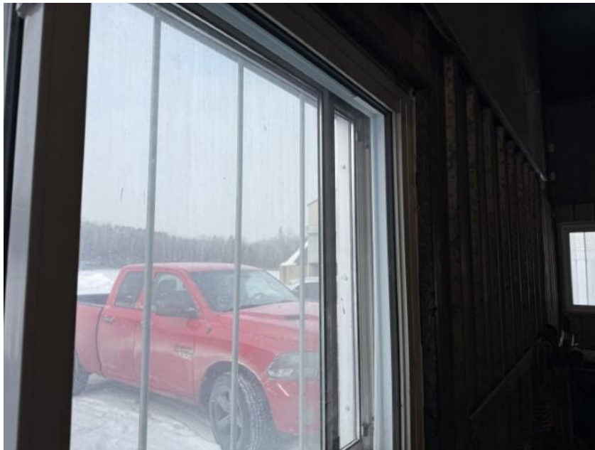
Photo 8: Municipal Garage – Overview of Interior Windows
